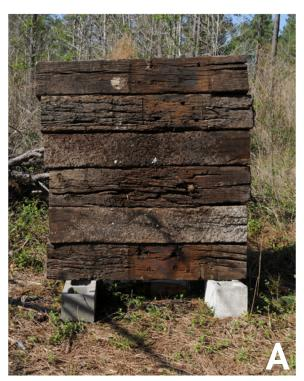
Space the left and right cinderblocks according to the width of the backstop you are constructing.
