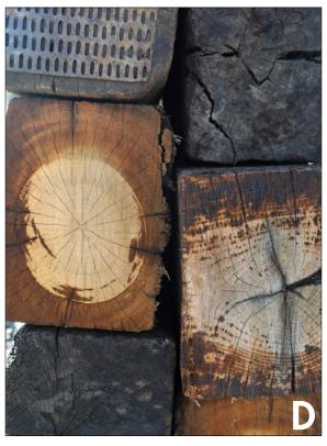
Cut the crossties in half and stack them two deep with the long side facing out. As you are stacking the crossties, make sure the seams of the back layer are offset from the front layer. This will prevent a projectile from passing through the backstop.
